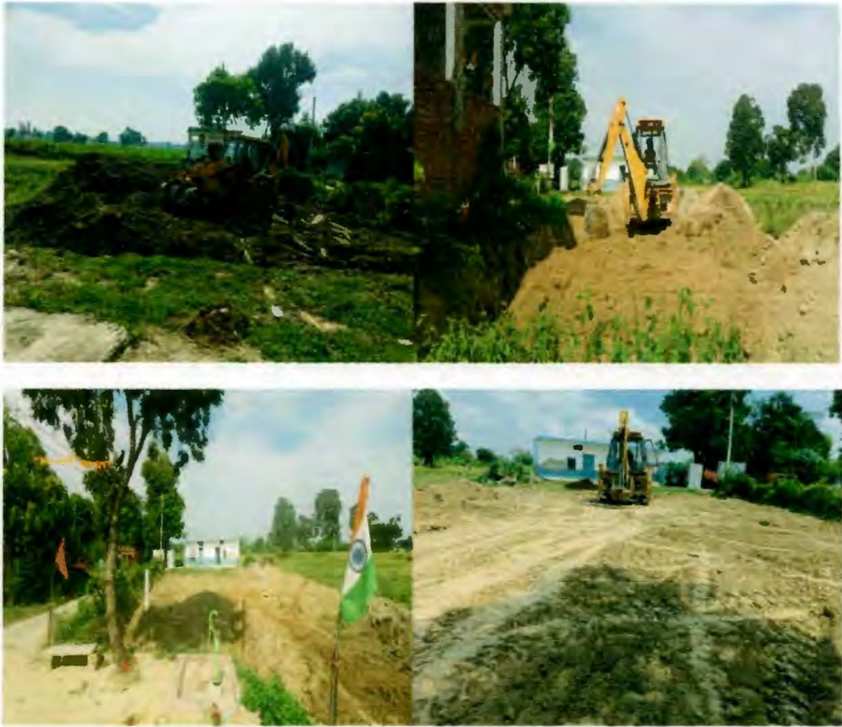
Fig- 10: Leveling Work
