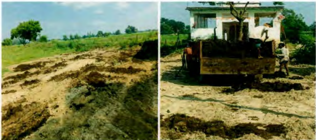
Fig- 11a: Mixing of Perforators, Water Retainers, Fertilizers & Micro-organisms
